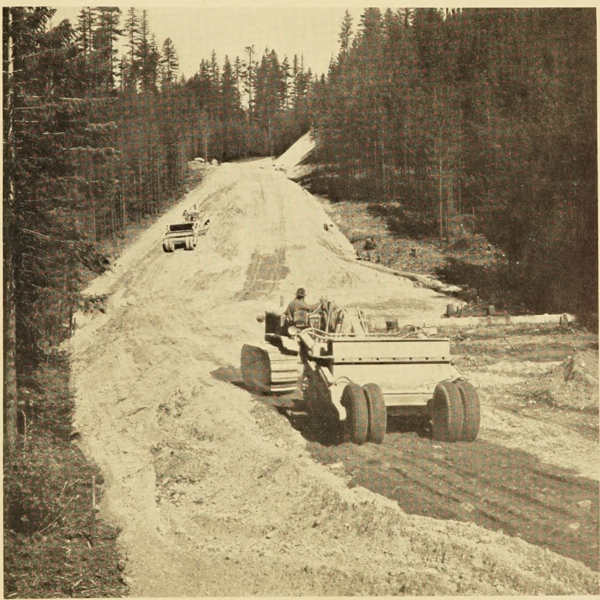
HIGHWAY FILL CONSTRUCTION OPERATIONS
